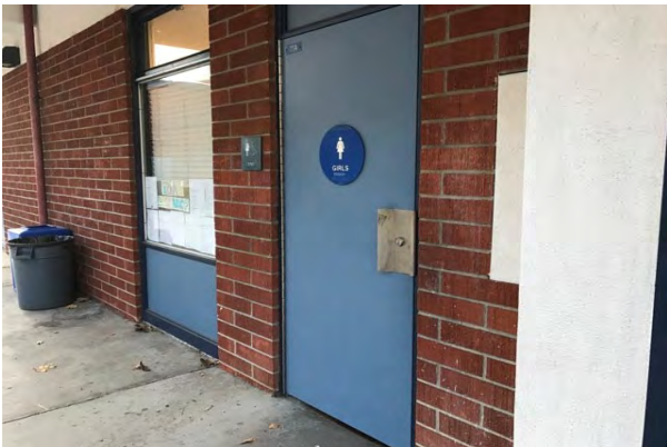
#17 STEEL EXTERIOR DOOR
