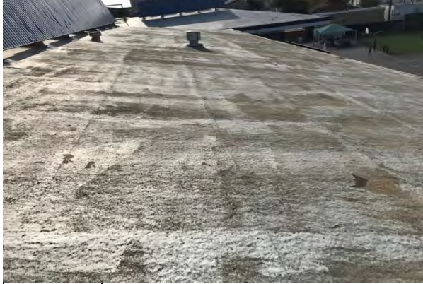
#19 BUILDING 3 BUILT-UP ROOF
