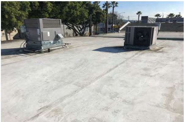
#18 SINGLE-PLY TPO/PVC MEMBRANE
