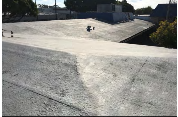
#20 BUILDINGS 1, 4 AND 5 BUILT-UP ROOFING
