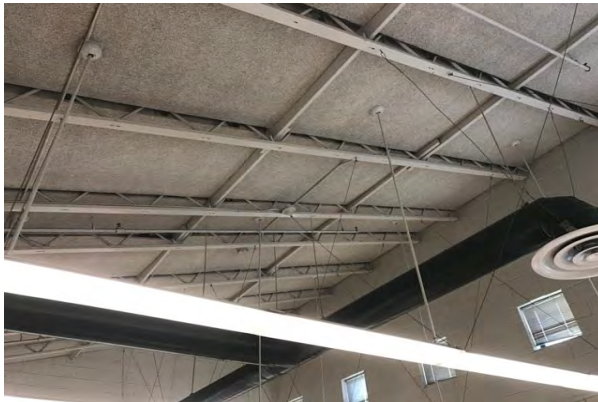
#9 BUILDING 6 STEEL FRAMED STRUCTURE
