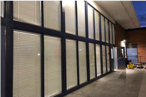
#15 STOREFRONT METAL-FRAMED WINDOWS
