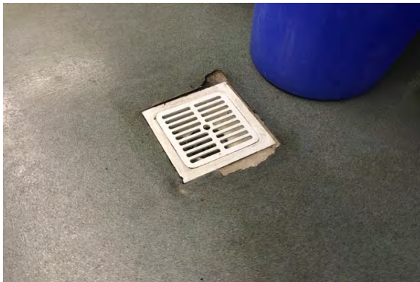
#35 CHIPPING EPOXY COATING
