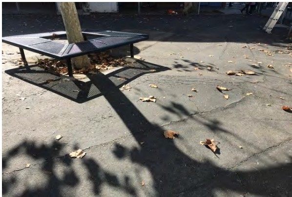
#65 LIFTING ASPHALT
