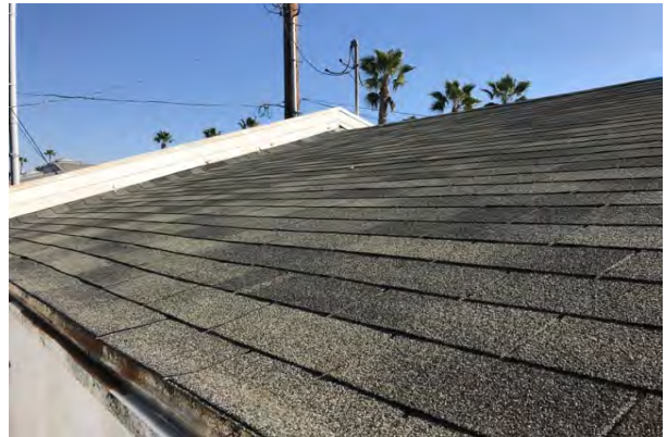
#22 BUILDING 10 ASPHALT SHINGLE ROOF
