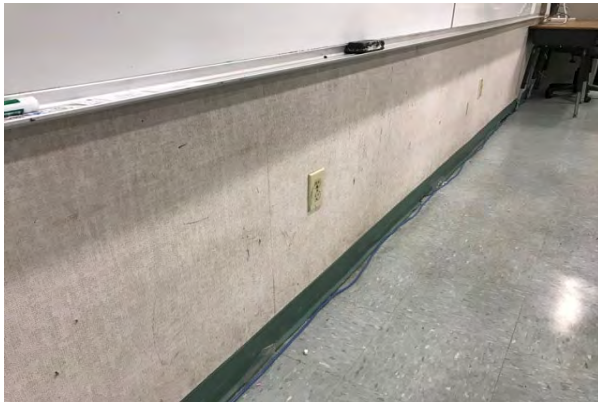
#33 PORTABLE BUILDING VINYL WALLS
